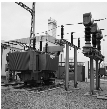
Fig. B14 : Air-breathing conservator-type tank at atmosphere pressure
